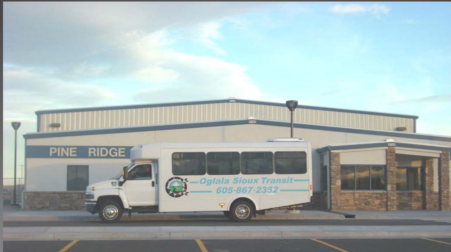
Oglala Sioux Nation Transit Facility
